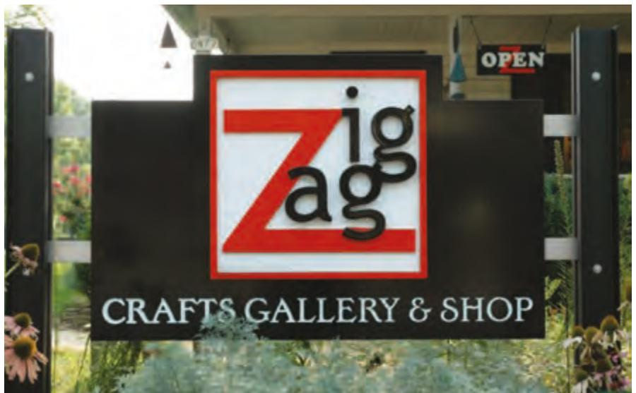
Carved Extria backer panel with raised/applied HDU logo panel. Posts are double steel c-channel with exposed stainless steel hardware for fun.
